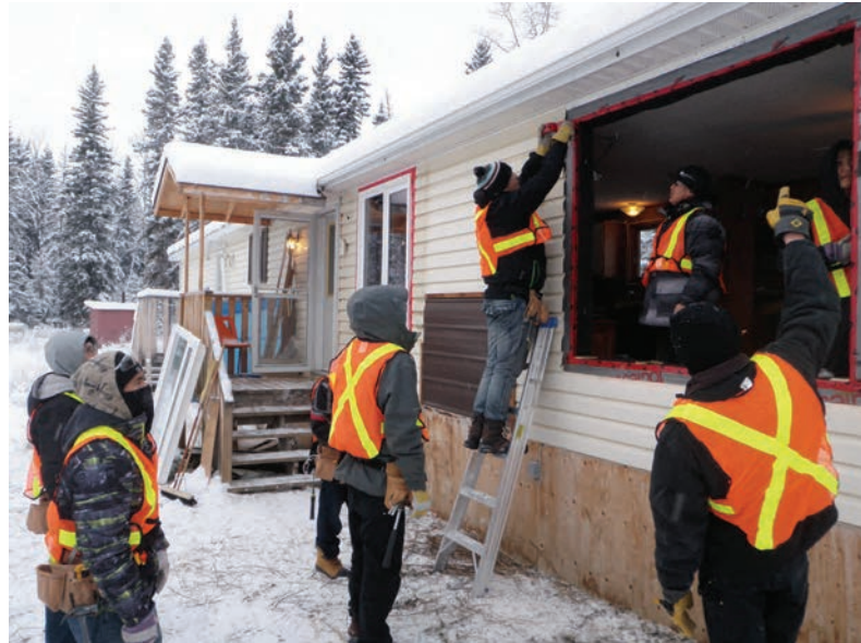
Students working hands-on replacing windows
